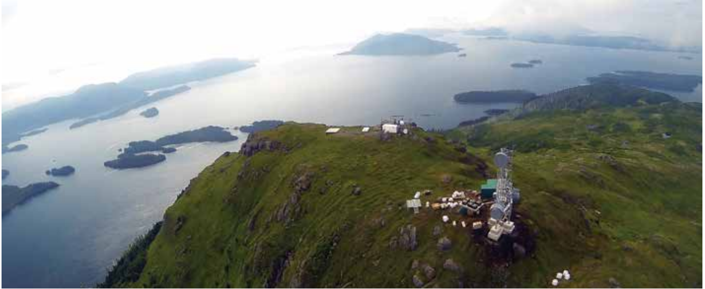
AP&T's Ketchikan crew completed a new 60-foot self-supporting tower and adjoining facilities hut on Sunnahae Mountain, located on Prince of Wales Island. The Sunnahae tower provides a new 1 Gbps link to AP&T's High Mountain site, and a downlink to the community of Klawock.
