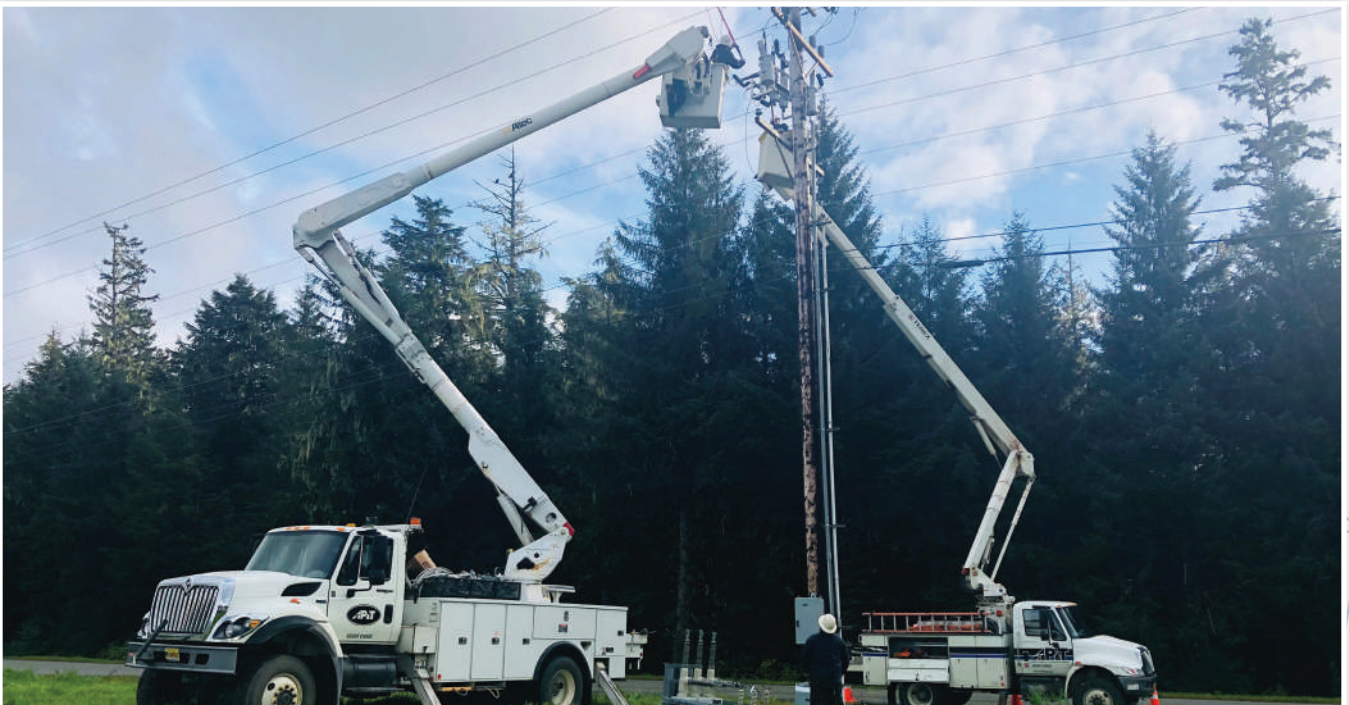
AP&T crews complete 'hot stick' work, performing maintenance without need for temporary outages.
